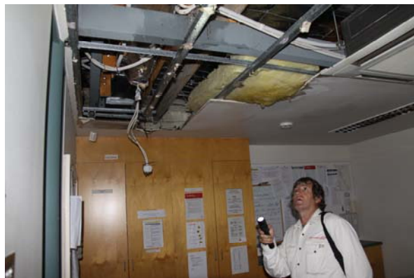
Water damage in the Wonambi Fossil Centre at Naracoorte. Photo: Steve Bourne.
